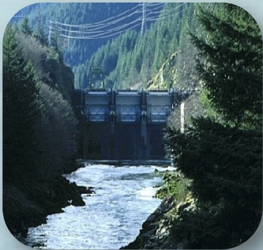
Big Cliff Dam, N. Santiam River, Oregon USA
