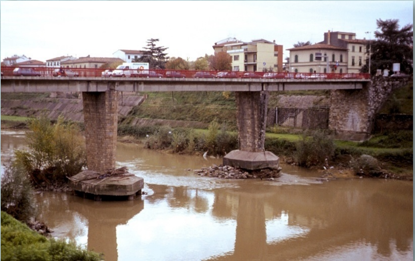
Channel incision and bed degradation Arno River at Empoli, Italy
